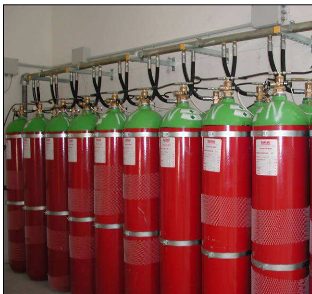
Fig. 3.3 Examples of system installation in single and double row configuration
