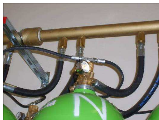
Fig. 3.39 Valve connections and discharge flex hose installation
