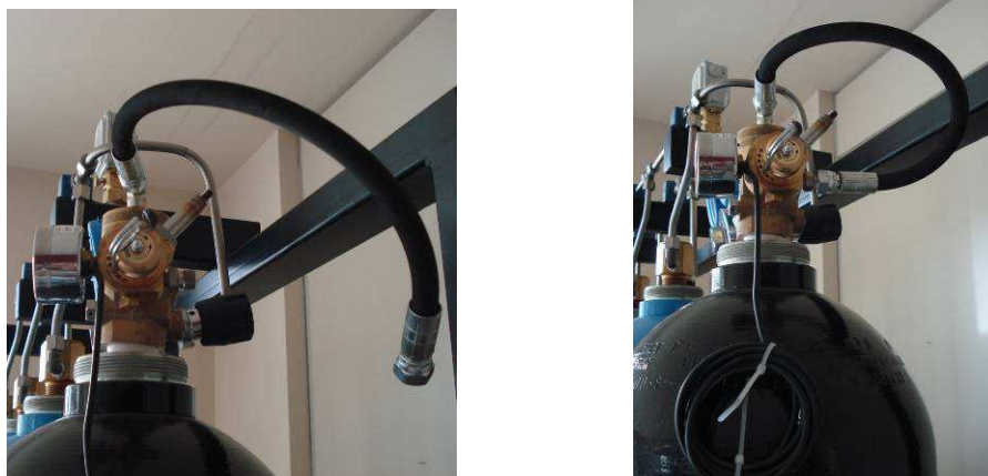
Fig. 7.1 Flex hose connection
