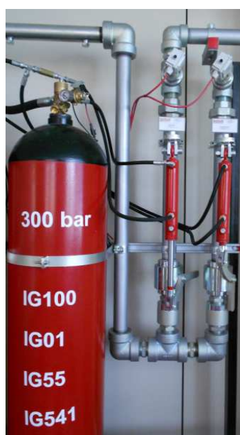
Fig. 2.33 Example of a 2 directional valves system
