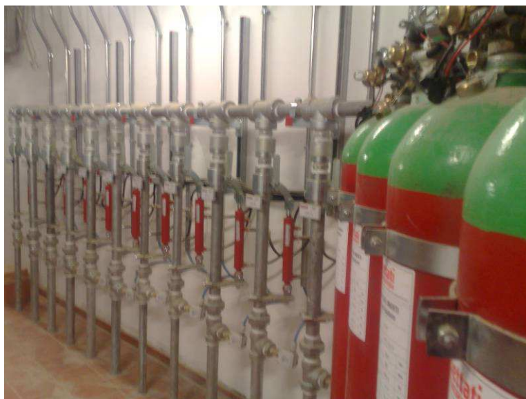
Fig. 2.5 Inert gas extinguishing system with directional valves
