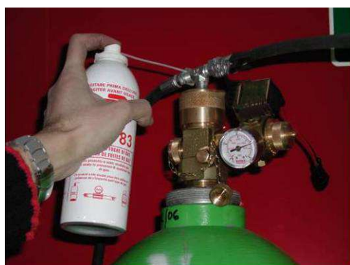
Fig. 5.5 Pneumatic circuit check (step 4, leak detection)
