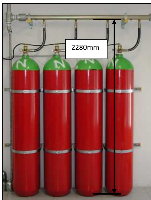
Fig. 3.1 Distance between manifold and floor level
