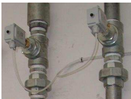
Fig.4.5 Pressure switch
