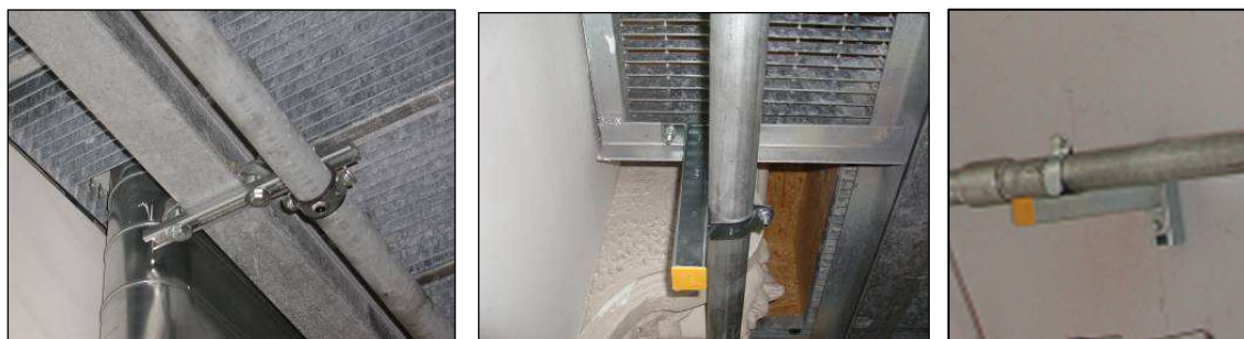
Fig. 3.48 Pipeline support systems
