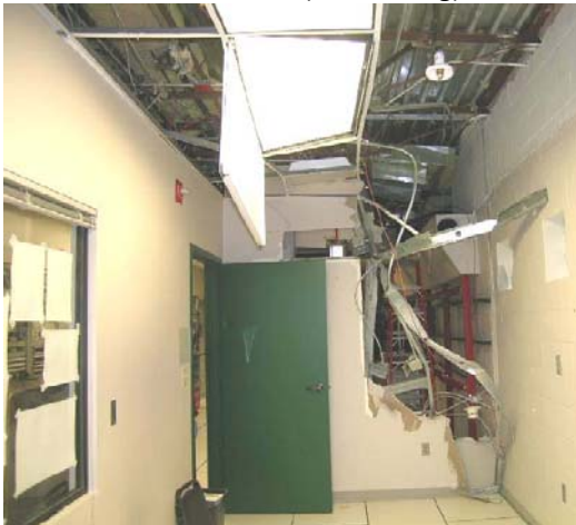
Fig. 4: An example of a high pressurization of the enclosure volume.
