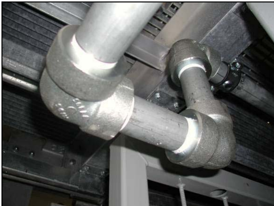
Figure 4.2 Piping system fittings
