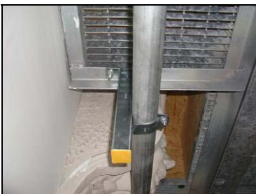
Figure 4.1 Piping system supports
