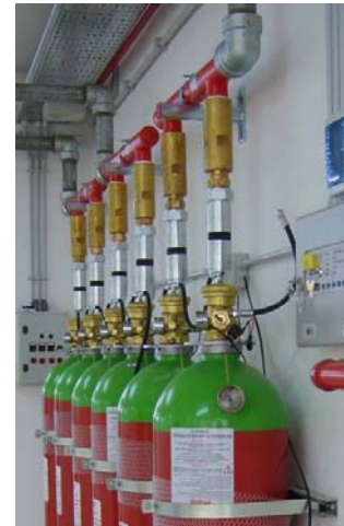
Figure 3.10 Manifold installation
