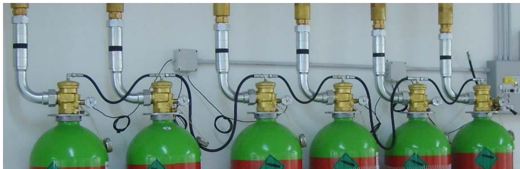
Figure 3.22 Pilot pneumatic connection
